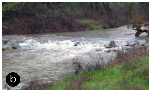
Figure 123—Flow redirection or training measures used to protect streambanks and structures, such as spur dikes or rock vanes (a), and rock drop structures or weirs (b). (Photos courtesy of John McCullah.)
