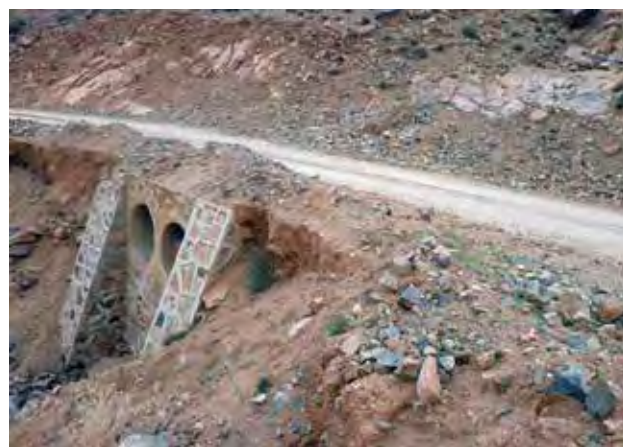
Figure 81—Culverts that have plugged due to their location in sediment and debris laden channels in a semiarid region.
