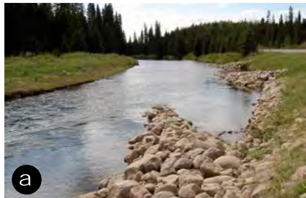
Figure 122—Ballested logs slowing the water along the bank during high flow in 2004 along State Route 542, Washington (a). Same location at low flow in 2011 (b). Note the streambank erosion in the riprap (in 2004) that took place before installing the ballested logs. (Courtesy of Roger Nichols.)
