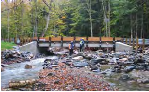
Figure 43—A bridge with minimum freeboard and located on an alluvial fan that nearly failed due to a log jam and subsequent aggradation in the channel. This forced some flow around the left abutment of the structure. (Courtesy of Bob Gubernick.)
