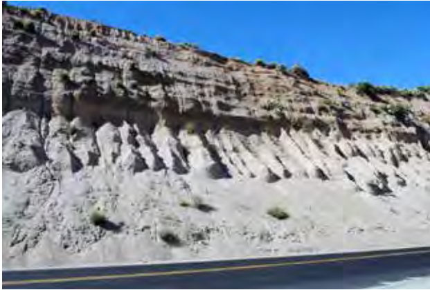
Figure 45—Severe erosion in a road cut slope in erodible soil. (Courtesy of Vincent Barandino.)
