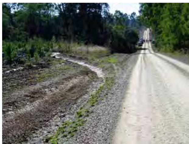
Figure 25—A leadoff ditch discharging into the forest before reaching a live stream at the bottom of the grade (near the parked vehicles).
