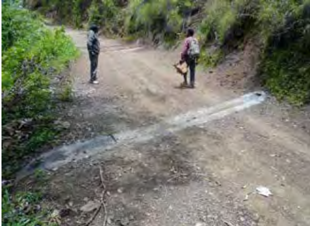
Figure 66—Small concrete channels placed across a native surfaced road for surface drainage. (Courtesy of Simon Done, TRL.)
