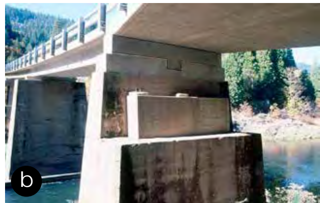
Figure 109—A bridge with marginal freeboard (a) where the abutments and piers were raised (b) to add freeboard and flow capacity, Plumas County, California.
