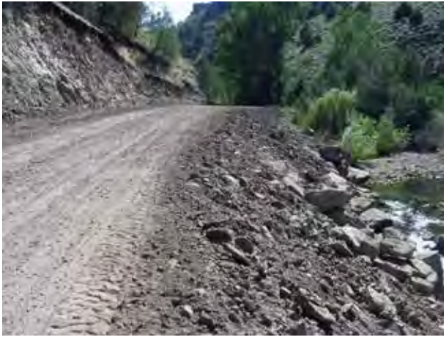
Figure 147—Road centerline is shifted away from the river after reconstruction, with a flatter, stable fillslope and riprap armor along the river. (Courtesy of Mike Balen.)
