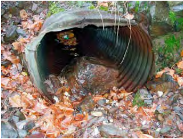
Figure 74—Damaged culvert inlets that need repairing and cleaning. Damaged culvert inlets can greatly reduce the culvert flow capacity.
