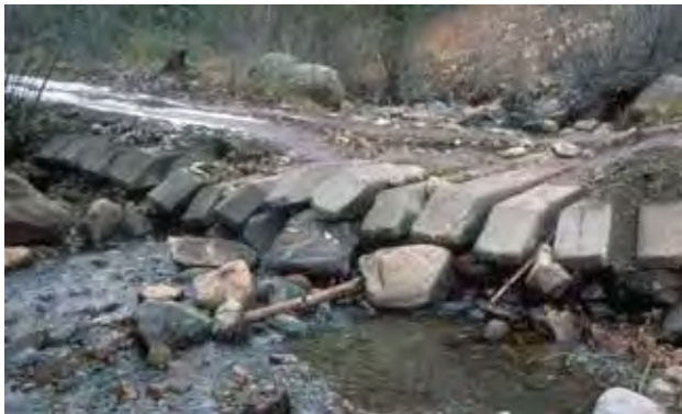
Figure 6—Damage to a low-water ford caused by scour of the bedding material under concrete planks.
