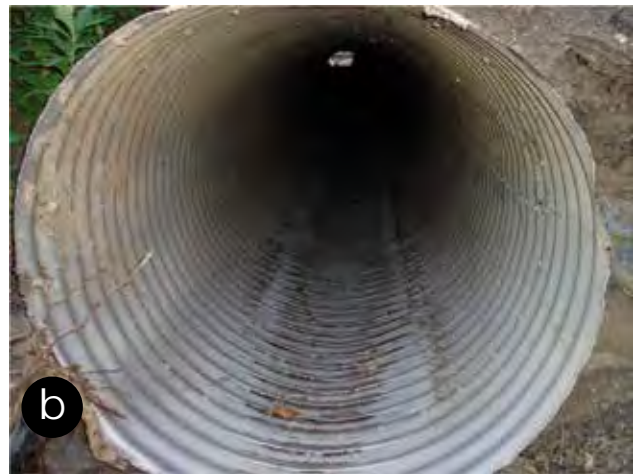
Figure 80—Problematic culverts due to piping under the structure (a) or deterioration from a worn-out bottom (b). These culverts are at risk of failure, particularly during a major storm event.
