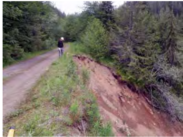
Figure 56—Road fill failure in a sliver fill that was partially supported by old logs. The failure triggered a downslope debris slide, Olympic National Forest. (Courtesy of Bill Shelmerdine.)
