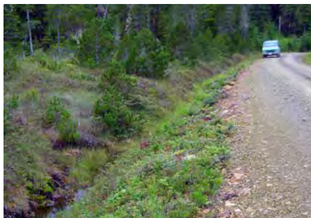
Figure 30—A ditch lined with vegetation (grasses). Note that as the ditch gradient increases the grasses alone may not be enough to prevent higher water velocities from eroding the ditch.
