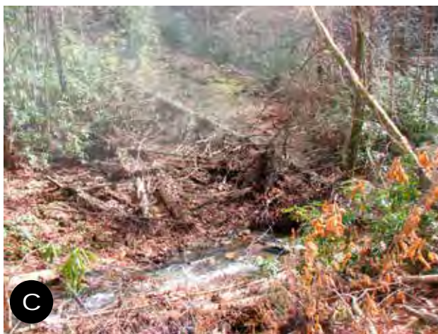
Figure 153—Examples of road closure treatments including a decommissioned road (a), an obliterated road and recontoured area (b), and closure of a road-stream crossing (c). (Lower photo courtesy of James Jones.)
