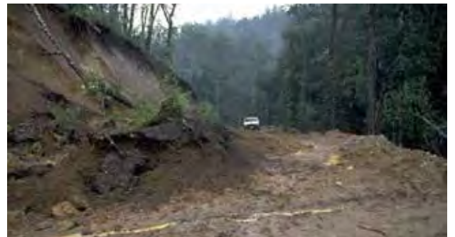
Figure 7—Culvert plugging (a) and a total culvert washout (b) during major storm events.
