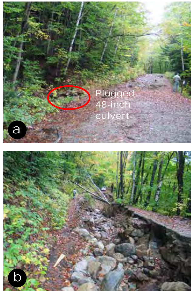
Figure 35—Stream diversion caused by a plugged 48-inch corrugated metal pipe that forced water down the road (a) and caused the roadway fill washout (b) when it exited the road, White Mountain National Forest. (Courtesy of Bob Gubernick.)
