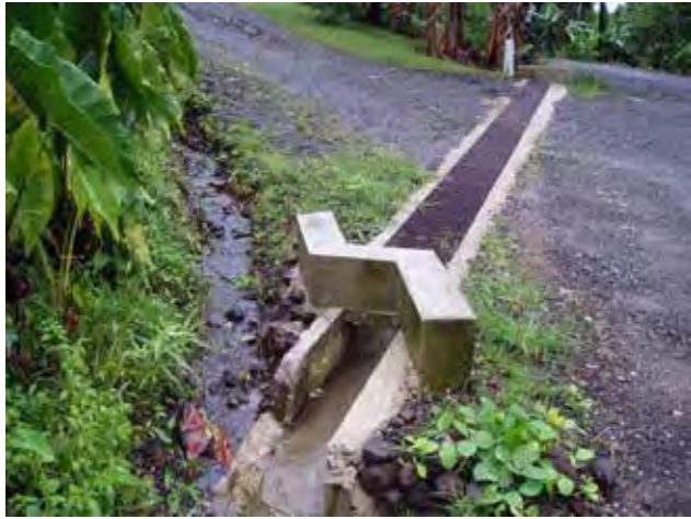
Figure 63—A relatively wide concrete open-top culvert with a metal grate.
