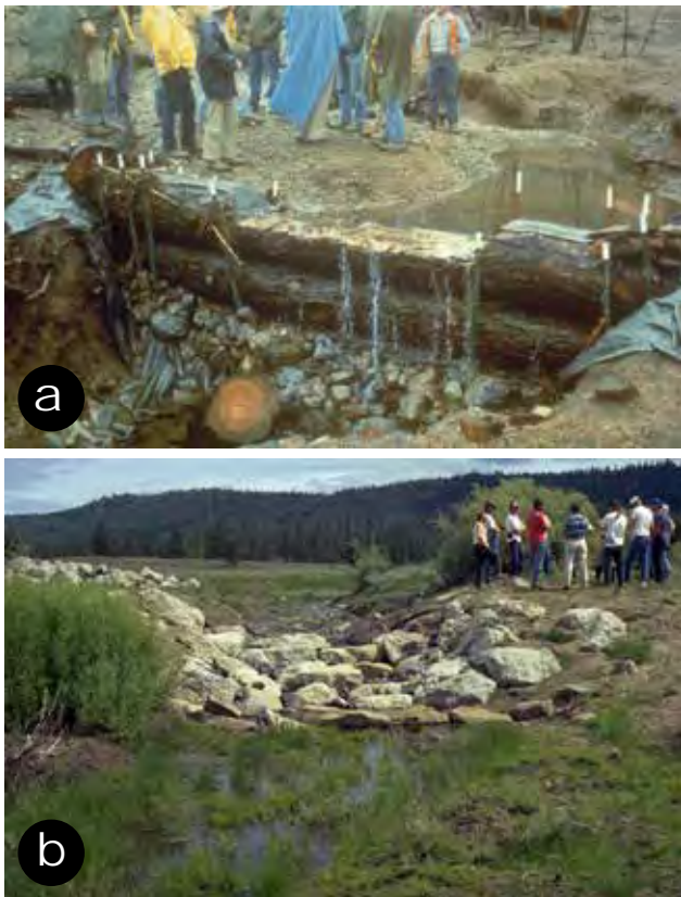
Figure 124—Gully stabilization structures made of logs (a) and of loose rock (b).
