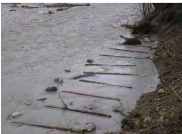
Figure 120—Warnick Bluff floating log weirs at high flow. Note the turbulent flow zone located outside the weir installation and slack water within the structure. (Courtesy of Roger Nichols.)
