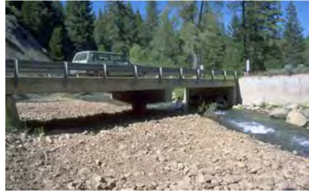
Figure 42—A bridge with significant channel aggradation on left from a growing point bar on the inside of a river bend that now needs removal to maintain bridge flow capacity. The point bar will rebuild with time, creating a continual maintenance problem at this bridge site. Bends are often poor locations for bridge sites.
