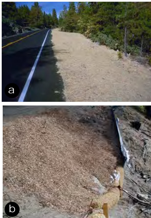
Figure 46—Common physical erosion control measures, including straw (a), netting, wood chips and straw wattles (b), to provide ground cover until vegetation can grow.
