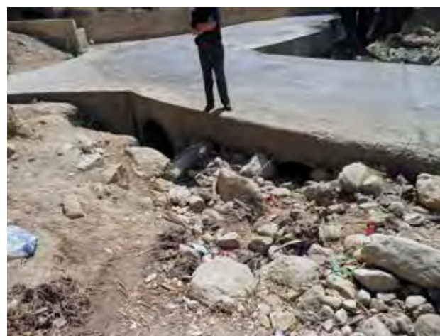
Figure 82—Culverts in vented low-water crossings that have totally or partially plugged with coarse channel debris.
