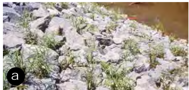
Figure 101—Rootwads, logs, and boulders (a) and brush layering (b) used for streambank stabilization (Upper photo courtesy of John McCullah).
