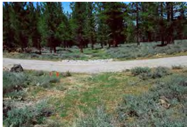
Figure 91—A simple rock-armored ford in an ephemeral channel. Coarse rock is placed across the channel bottom and a fine aggregate is placed on the road surface for driver comfort.
