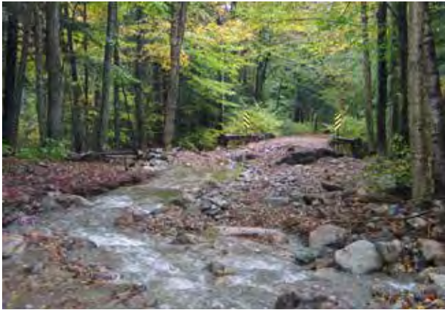
Figure 37—Stream diversion down a road caused by stream aggradation that filled the channel and plugged a bridge. (Courtesy of Bob Gubernick.)
