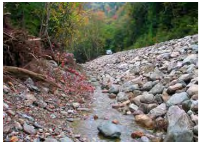
Figure 98—A stream with light riprap armoring on the roadway fill, but the channel bottom is not armored, nor is the toe of the riprap slope keyed into the channel below the depth of potential scour. This site is likely to fail in a future storm. Also the channel is constricted. Road relocation should be considered here. (Photo courtesy of Bob Gubernick.)
