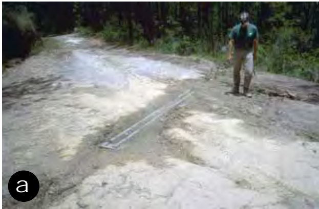
Figure 63—A relatively wide concrete open-top culvert with a metal grate.
