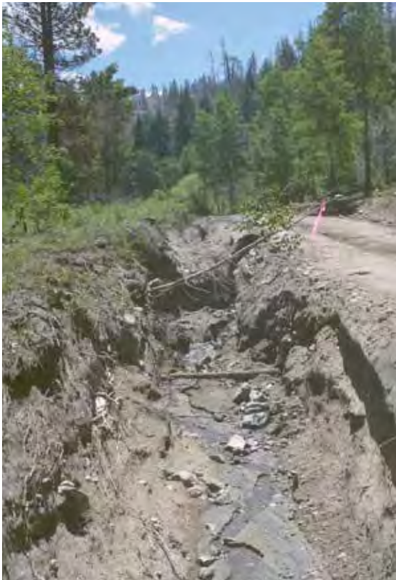
Figure 2—Severe gully erosion damaging forest roads during storm events.
