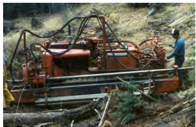
Figure 137—Horizontal drains being drilled to drain groundwater and stabilize a large landslide.
