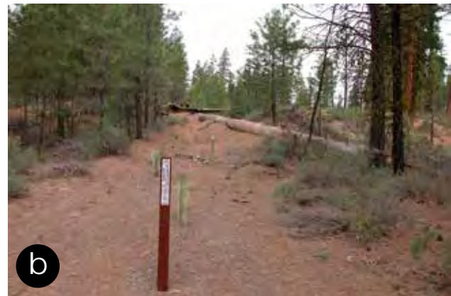
Figure 154—Examples of roads that have been placed into storage. Photo (a) shows a road that has been closed using a waterbar. (Courtesy of Ken McCall/Karen Bennett.) Photo (b) shows the road has been closed with a log and berm, plus some vegetation. (Courtesy of Greg Napper.)
