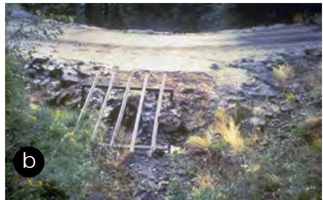
Figure 77—Use of trash racks to prevent plugging of a culvert or bridge from upstream large boulders and debris. (Bottom photo courtesy of Vincent Barandino.)
