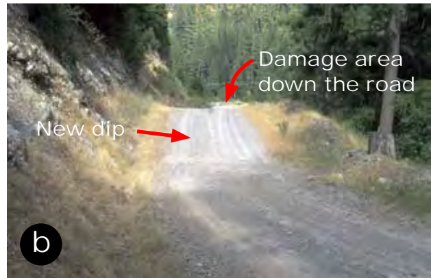
Figure 39—Another storm damage diversion site with road damage down the road at the curve (a) and the diversion-prevention dip added up the road above the damaged area (b) just below the culvert crossing (not seen in photo) to prevent future stream diversion, Plumas National Forest.
