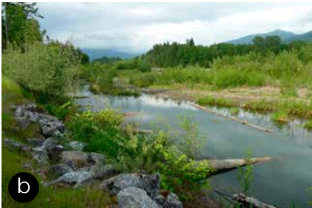
Figure 122—Ballested logs slowing the water along the bank during high flow in 2004 along State Route 542, Washington (a). Same location at low flow in 2011 (b). Note the streambank erosion in the riprap (in 2004) that took place before installing the ballested logs. (Courtesy of Roger Nichols.)
