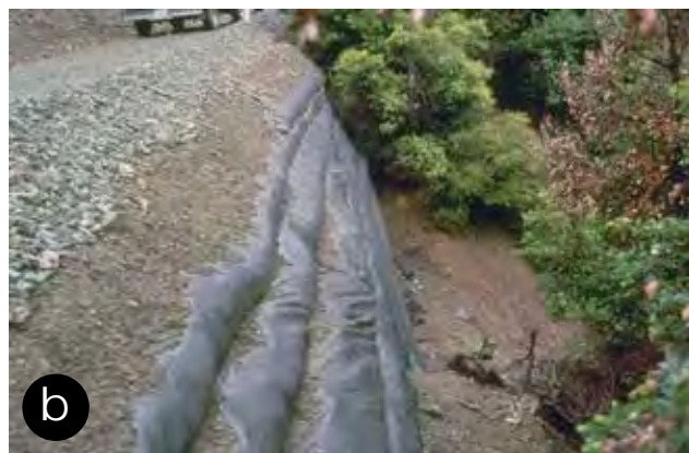
Figure 133—A welded wire MSE wall (a) and a geotextile wall (b), both used because of their relatively low cost and ease of construction.
