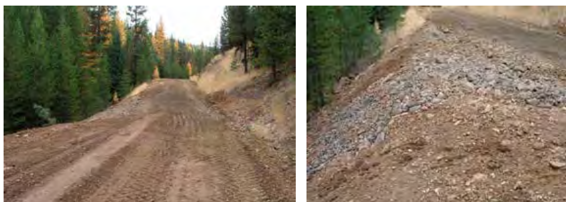
Figure 17—An armored and grid-rolled rolling dip on the Umatilla National Forest. Note the armored dip outlet using small riprap. (Courtesy of Caty Clifton, Umatilla National Forest.)
