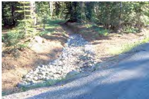
Figure 22—A cross-drain culvert with an armored outlet and leadoff ditch on fairly flat ground.
