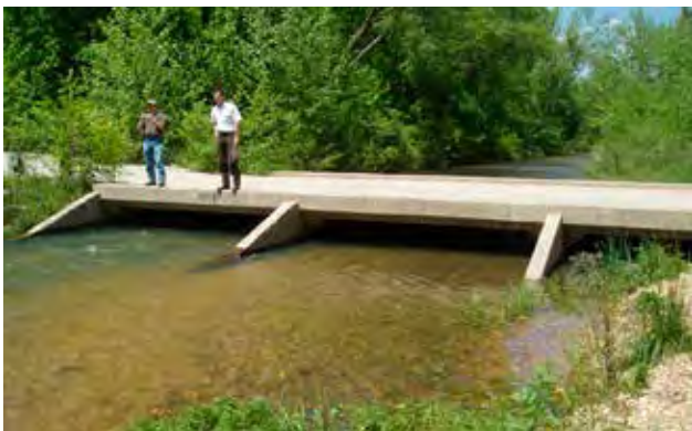
Figure 90—A large vented low-water crossing with predominantly natural stream channel bottom material that is ideal for fish passage.
