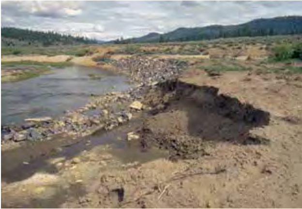
Figure 9—Streambank erosion during a major flood and loss of riprap streambank stabilization material. Surrounding land management contributes to the susceptibility of a road to damage. In this instance, grazing practices and poor riparian conditions (compacted soils devoid of deep-rooted vegetation) contributed to severe streambank erosion. Poor installation and undersized riprap contributed to the problem.
