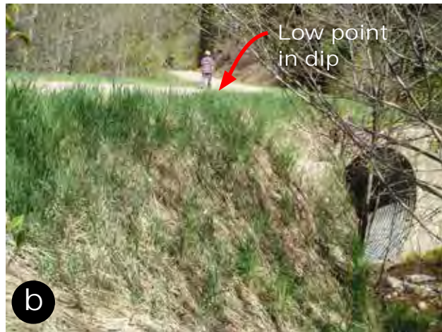
Figure 38—A concrete headwall (a) and an overflow dip placed just down the road (as seen at the low point where the person is standing down the road (b)) to prevent future stream diversion. This is the culvert repair and diversion-prevention dip installed at the damage site seen in figure 34.
