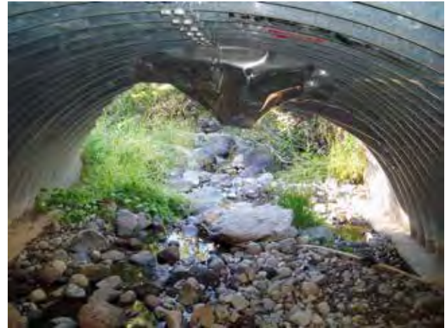
Figure 74—Damaged culvert inlets that need repairing and cleaning. Damaged culvert inlets can greatly reduce the culvert flow capacity.
