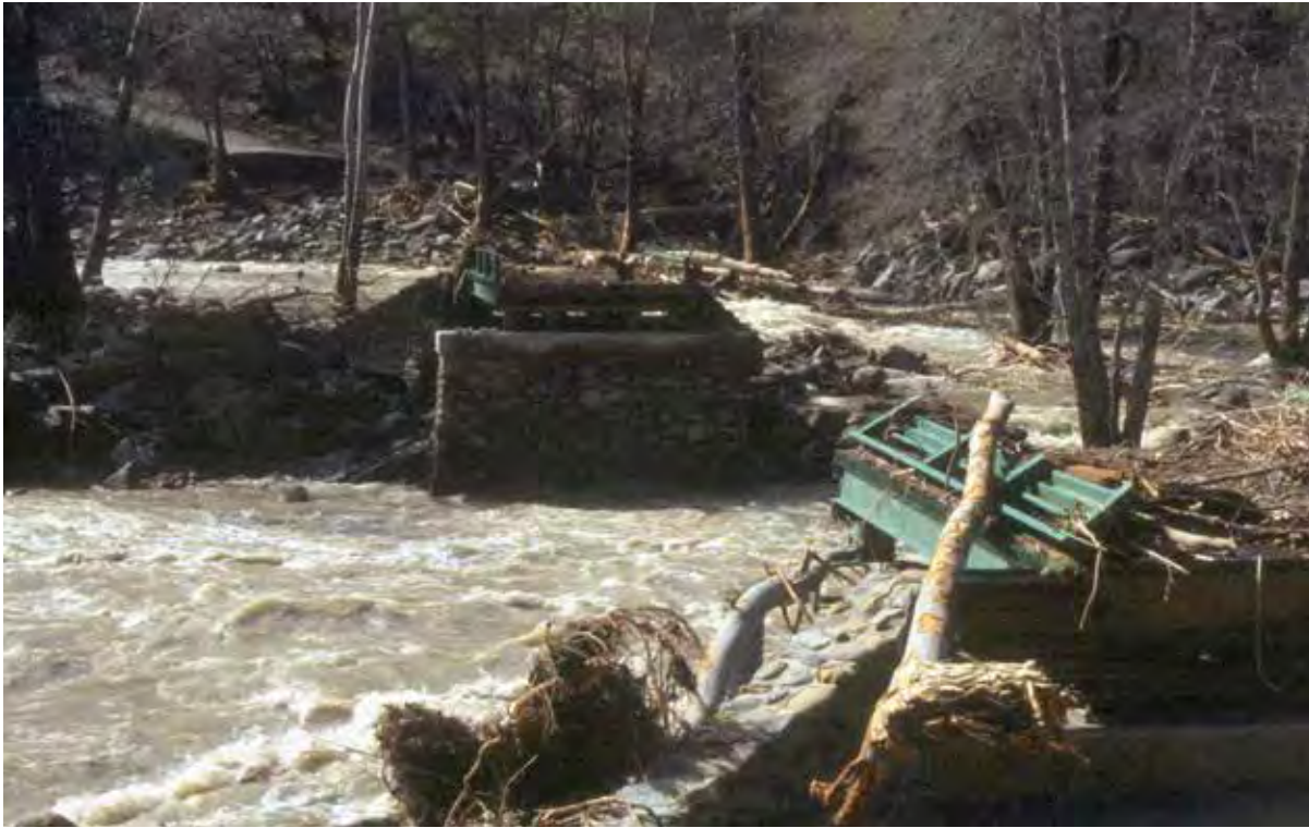
Figure 108—A failed bridge due to lack of freeboard and accumulation of debris behind the bridge deck.
