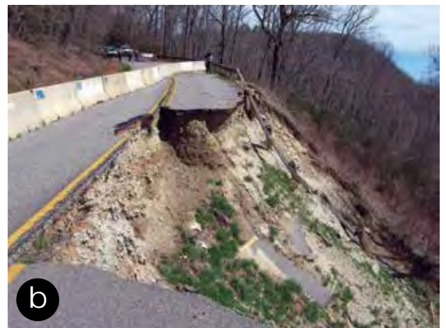
Figure 58—Debris slides that subsequently formed gullies below the road in Colorado (a) and on the Blue Ridge Parkway, Pisgah National Forest, North Carolina (b). (Lower photo courtesy of Tom Collins.)
