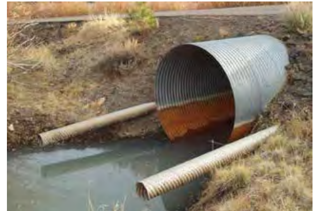
Figure 105—Perforated pipes flowing through or next to larger main pipes to maintain some flow through the pipe even with beaver dam activity.
