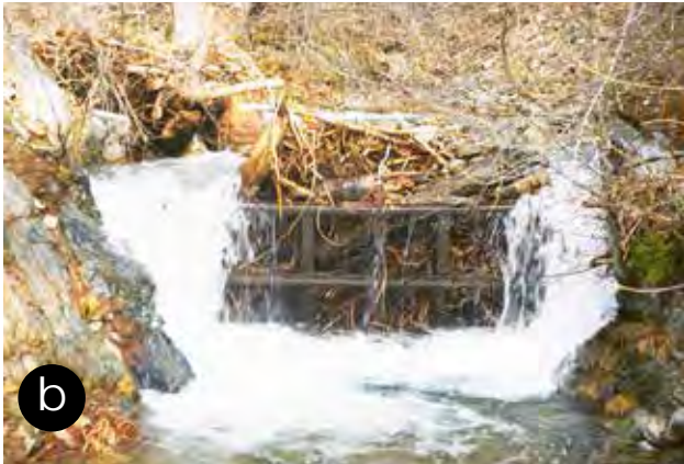
Figure 79—A trash rack upstream of a culvert, both before a storm ((a) looking downstream) and full of debris after a major storm event ((b), looking upstream). Note that trash racks must be cleaned and maintained!
