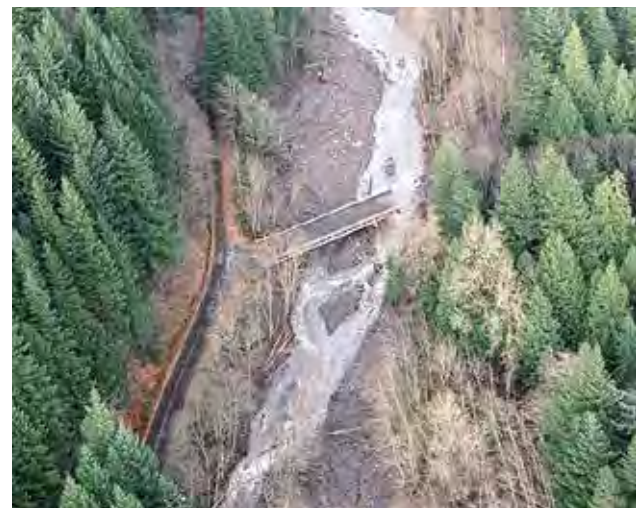
Figure 4—A bridge abutment washed away by a debris torrent and channel widening during a storm event in the Pacific Northwest. (Courtesy of Mark Levertton.)
