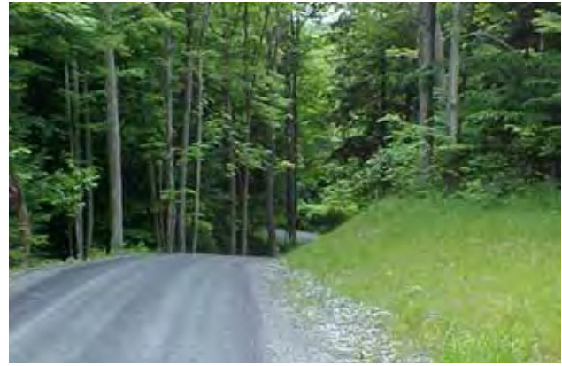
Figure 139—A variety of vegetation used to stabilize cutslopes. Selection of vegetation type depends a great deal on the local climate and environment, but deep-rooted species are critical to achieve slope stabilization. (Right photo courtesy of the Pennsylvania State University Center for Dirt and Gravel Road Studies.)
