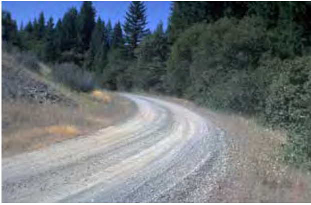
Figure 61—An outslope road template on a curve in the road. This photo also shows the tendency of a center and outside berm to form on gravel roads. The presence of these berms disrupts the dispersion of water and can cause significant water concentration if not eliminated by routine maintenance or dispersed with use of rolling dips.
