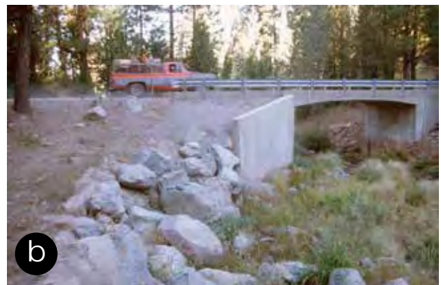
Figure 113—Abutment scour caused by channel meander (a) and the repair (b), extending bank protection upstream from the bridge. Note that the bridge also constricts the original stream channel, Plumas National Forest.
