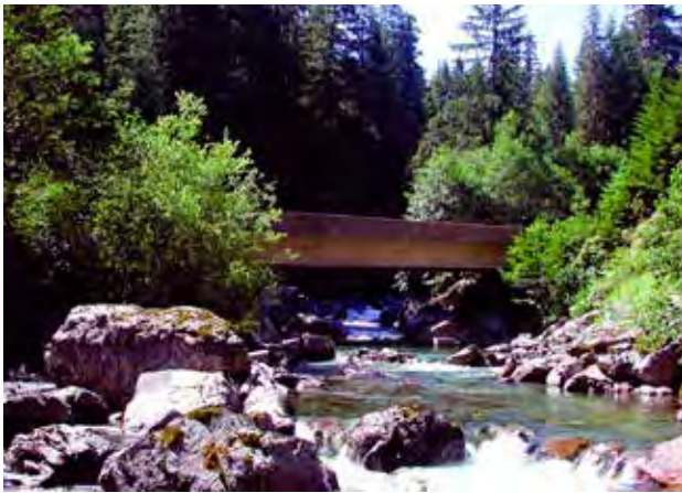
Figure 41—A bridge opening and channel relatively free of vegetation and debris.
