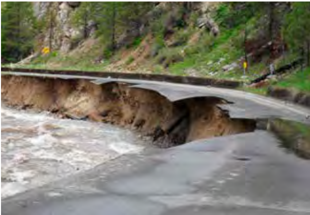
Figure 10—Road-stream encroachment and flooding along the South Fork, Salmon River, Idaho, due to a rain-on-snow event. (Courtesy of Tom Black.)
