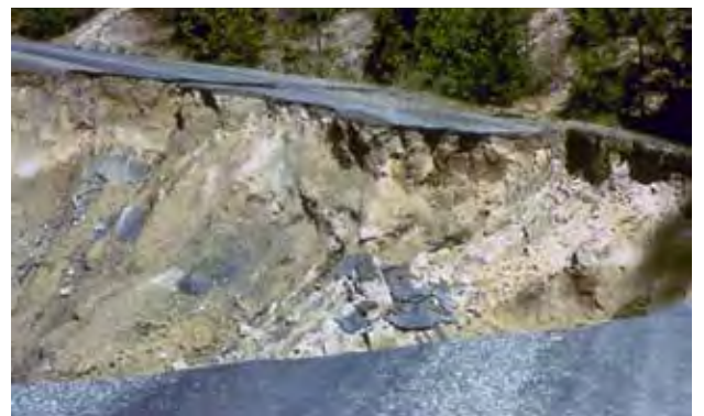
Figure 8—Examples of road closure caused by cutslope and fill failures during storms.
