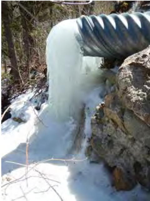
Figure 149—Iced culvert at milepost 2.5 on Mt. Washington Auto Road, NH. (Photo courtesy of the Mt. Washington Auto Road.)
