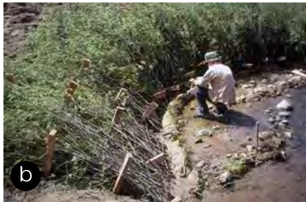
Figure 101—Rootwads, logs, and boulders (a) and brush layering (b) used for streambank stabilization (Upper photo courtesy of John McCullah).
