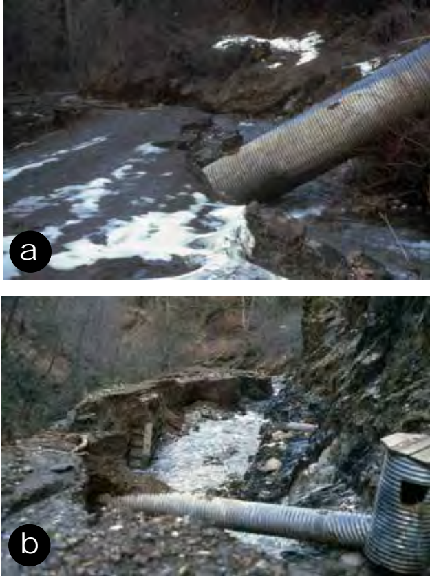
Figure 34—A plugged pipe that “floated” out of the fill (a), resulting in a stream diversion down the road and past a culvert cross drain with metal drop inlet, (b), causing extensive damage to the road and significant environmental impacts, Plumas National Forest.
