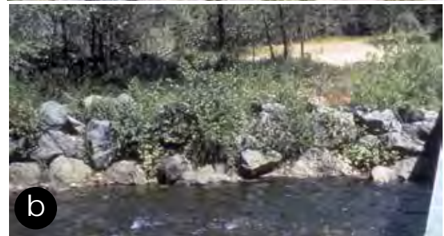
Figure 102—Biotechnical streambank stabilization using rock riprap and live willow stakes. (Photo (a) courtesy of Robbin Sotir.)
