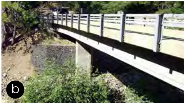
Figure 112—Bridges with rock riprap (a) and gabion (b) scour protection around the abutments since the bridges are located on bends in the stream (river bends are problematic locations).
