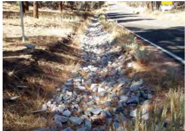
Figure 27—A rock armored ditch to control the waterflow and prevent downcutting of the ditch.
