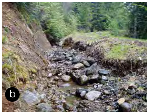
Figure 36—Stream diversion caused by plugging of a 48-inch culvert (a) and subsequent cascading failure and road damage on down the road (b), region 6, Washington. (Courtesy of Robin Stoddard.)
