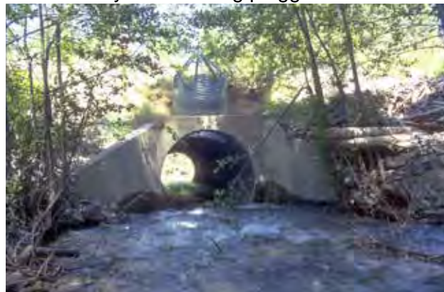
Figure 71—Culvert with a riser pipe and trash rack to prevent plugging in a channel that carries a lot of debris. Note that the roadway barely is seen in the background above the riser-pipe elevation.
