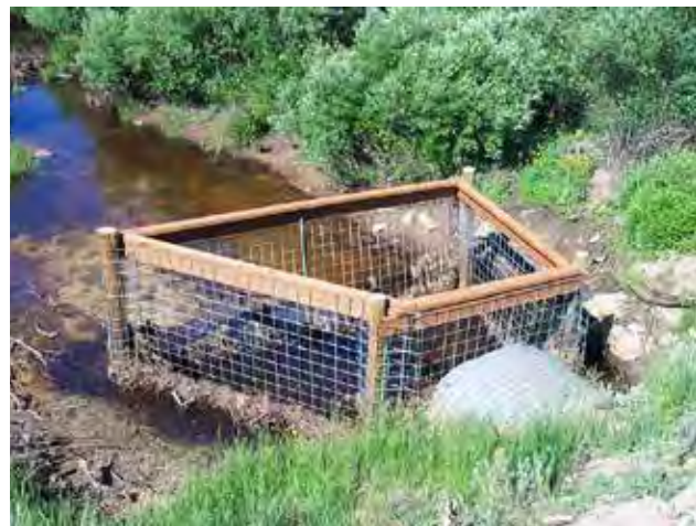
Figure 106—Beaver deceiver protection by screening off the entrance to the culvert in Wyoming. (Courtesy of Steve Coupal.)
