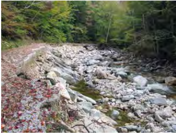
Figure 117—Road-stream encroachment where a road is located too near the stream in a narrow river canyon, confining the streamflow during a major storm event, Green Mountain National Forest. (Courtesy of Bob Gubernick.)
