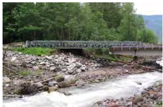
Figure 114—Channel widening and scour around a bridge abutment, removing part of the approach fill, caused by a debris torrent and shifting river channel. A temporary Bailey Bridge is being used to cross the gap, Mount Hood National Forest. (Courtesy of Mark Leverton.)
