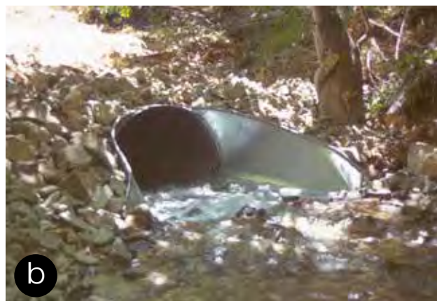
Figure 70—Culverts with a concrete headwall (a) and a metal end section (b) that offer improved resistance to plugging and damage from overtopping.
