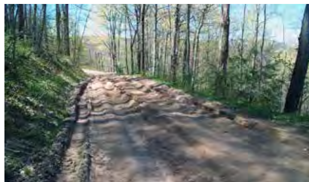
Figure 12—Ruts and erosion in the road surface because of lack of surface drainage and maintenance. This road in this condition is particularly susceptible to damage from any storm. (Photo courtesy of Vincent Barandino.)
