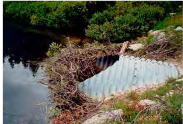
Figure 103—A beaver dam partially plugging a large culvert, Routt National Forest. (Courtesy of Steve Coupal.)
