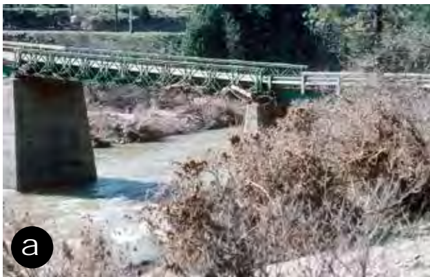
Figure 109—A bridge with marginal freeboard (a) where the abutments and piers were raised (b) to add freeboard and flow capacity, Plumas County, California.
