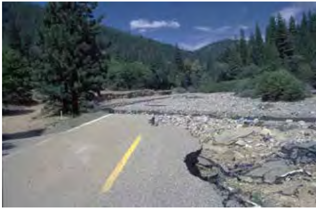
Figure 5—This road washed out because of placement on a flood plain and channel widening during a storm event.
