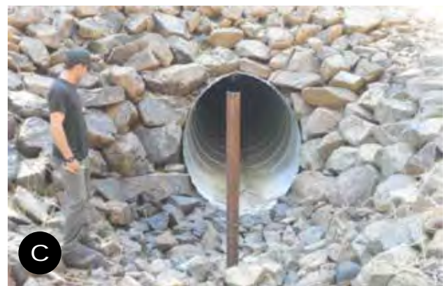
Figure 78—Examples of trash racks added to small culvert pipes to prevent plugging. Note that the riser with trash rack (a) is downstream of a fire area where considerable sediment is anticipated that often plugs small pipes. Debris can float over the culvert inlet at high flows (b). The single post (c) upstream of the pipe is used to help orient debris to go through the pipe rather than plugging across the inlet.
