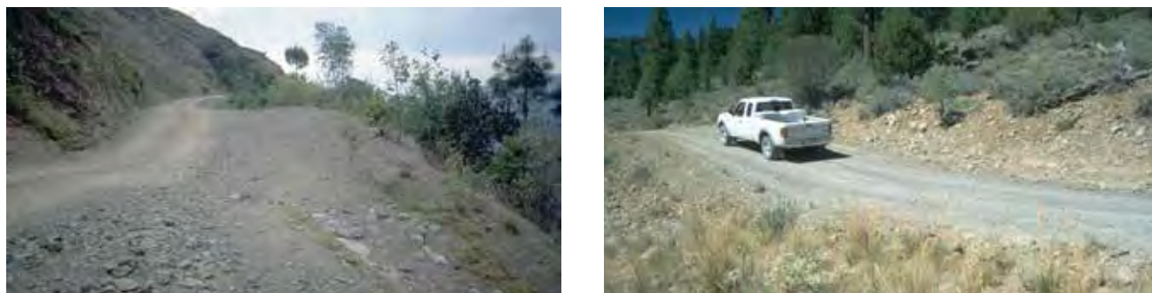
Figure 16—The form of rolling dip cross drains on various roads.
