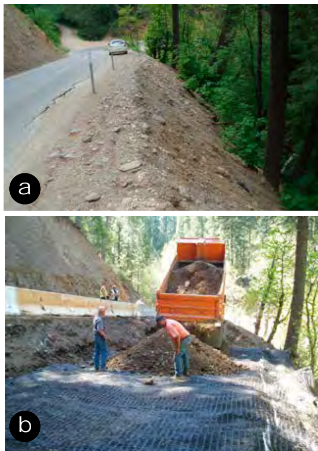
Figure 145—Over-steep settling fillslope before deep patch repair (a) and a geosynthetic reinforcing material (a geogrid) being placed in a deep patch shoulder repair (b).
