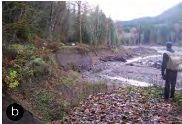
Figure 116—Examples of roads located in flood plains (a) and on the edge of a channel migration zone (b) where flood damage may be frequent and costly. Road access may be lost for long periods of time, Pacific Northwest. (Courtesy of Roger Nichols.)
