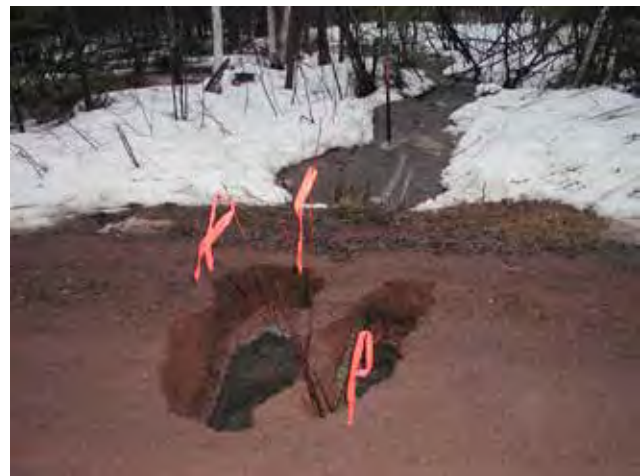
Figure 150—Culvert clogged with ice causing water to flow across the road. (Courtesy of Dale Higgins, Chequamegon-Nicolet National Forest.)
