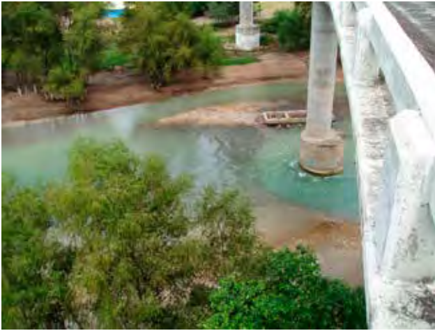
Figure 111—Common scour seen around a mid-channel pier or abutment. Thus mid-channel piers and abutments are problematic, undesirable, and should be avoided if possible.
