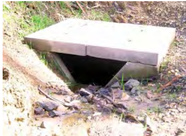
Figure 67—A variety of culvert cross-drain drop inlet structure types used on forest roads.
