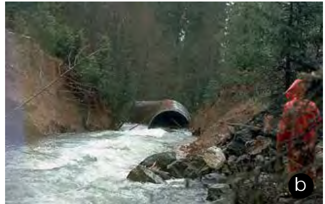
Figure 7—Culvert plugging (a) and a total culvert washout (b) during major storm events.
