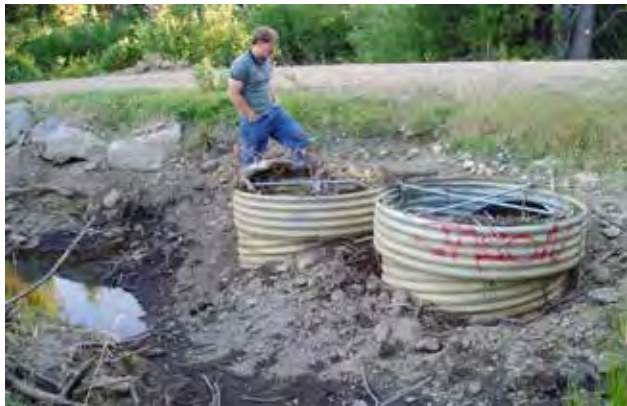
Figure 104—Large riser pipes connected to culverts with entrance rings to allow waterflow into the pipe, yet thwart beaver activity, Plumas National Forest, California.
