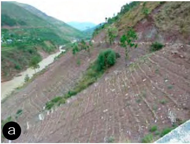
Figure 142—Before (a) and after one season (b) photos of brush layering used to stabilize an entire hillside after storm damage in Pakistan. (Photos courtesy of Asif Faiz, World Bank.)
