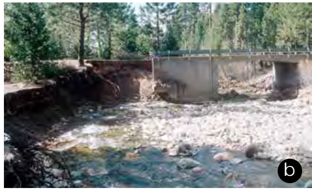
Figure 3—Bridge scour occurring at the abutment of bridges during major storms in northern California because of channel constriction (a) and natural stream meander (b).
