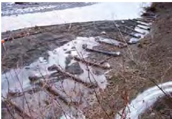
Figure 118—Floating log weirs just after installation. These weirs are designed to move the river thalweg away from the near bank, Warnick Bluff, Nooksack River, Washington. (Courtesy of Roger Nichols.)
