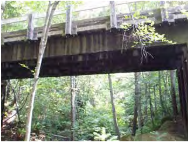
Figure 40—Stream channel under a bridge that needs clearing and tree removal if flows are being blocked, diverted, or if there is risk of plugging the bridge.
